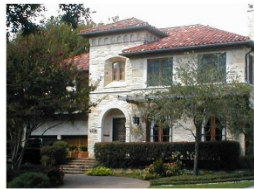
This two-story house has a prominent entry for the style with a tiled cornice for shading from sun exposure.
