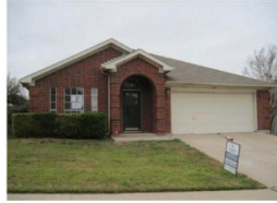
Brick windows are detailed improperly. The garage is too prominent in the elevation.
