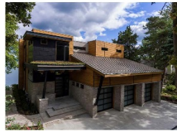
This contemporary home has a monoslope steel roof, exposed structural steel members and a covered carport.
