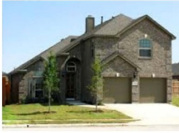
The garage is most prominent and creates disproportionate overall massing. Vent stacks are visible from the street.
