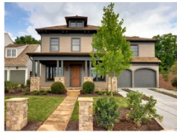
This home features a prominent porch with paired columns and a garage set back from the main body of the house.
