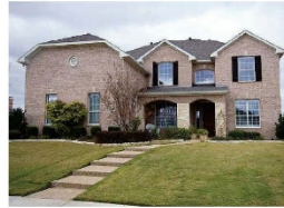
The garage on this home is the largest mass in the elevation. Sillars are not sized properly for the openings.
