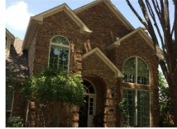
The openings are too large for the home. The massing is too complex for the width of the front facade.
