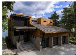
This contemporary house has a monoslope steel roof, exposed structural steel members and flat-topped patios.
