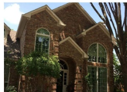
The coverings are too large for the house. The massing is too complex for the width of the front facade.
