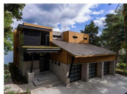
This contemporary home has a monoslope steel roof, exposed structural steel members and flat topped garages.
