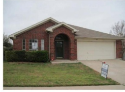
Entry windows are detailed improperly. The garage is too prominent in the elevation.
