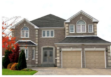
The window openings are too large and out of proportion for the façade. This house has a complex massing where the gable elements are competing for importance.
