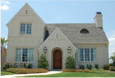
This house design has a gable set back from main house. Entrance is prominent. Massing is more complex with some variation. Minimal detailing is appropriate for the style.
