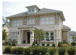
This craftsman-style home has added roof detailing and well-proportioned openings. The outdoor terrace helps to capture outdoor space.
