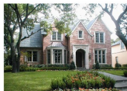
This house has well-detailed masonry openings with a prominent entrance and simple massing.
