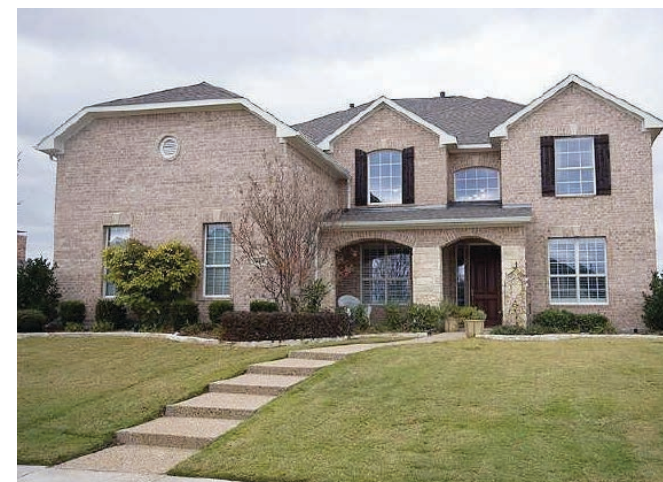
The garage on this home is the largest mass in the elevation. Shutters are not sized properly for the openings.
