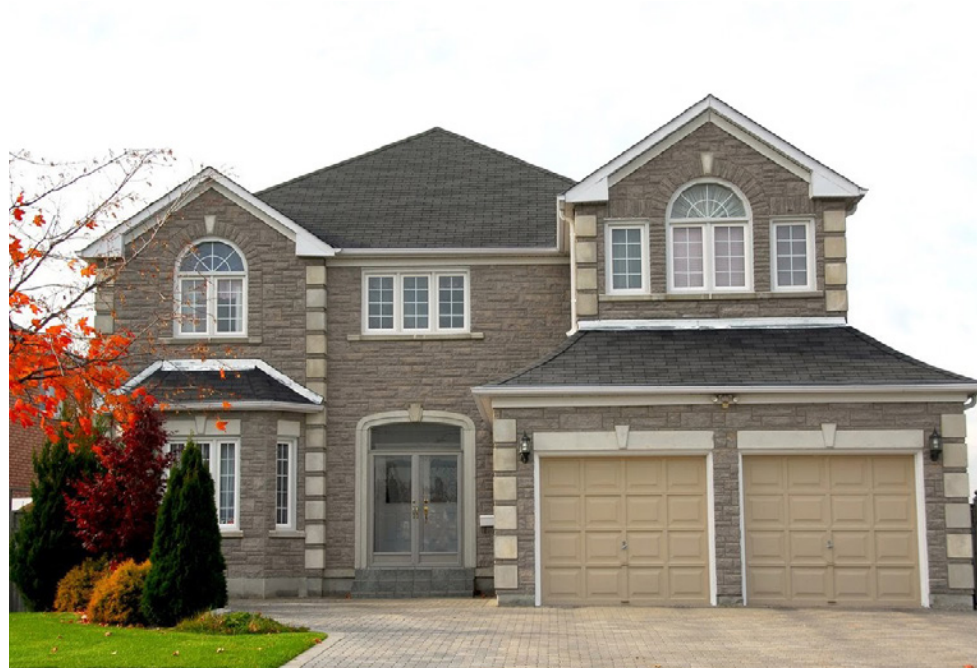
This home design has a prominent garage forward of the main house. The proportions and openings for this home are too small for the overall massing.
