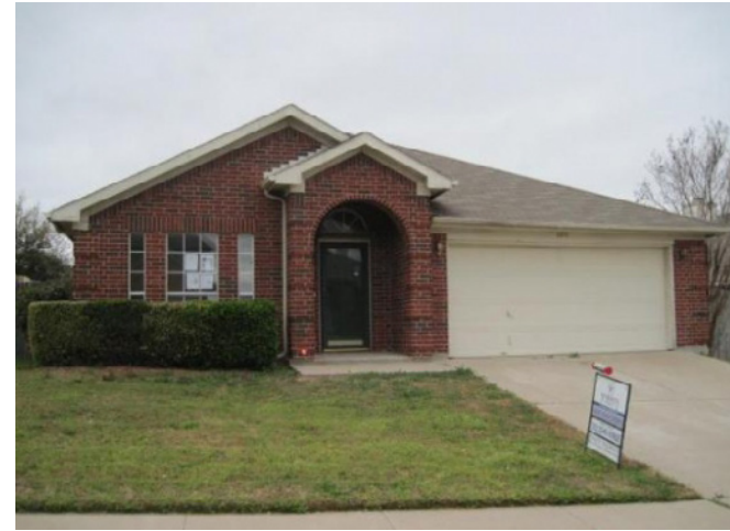
Paired windows are detailed improperly. The garage is too prominent in the elevation.
