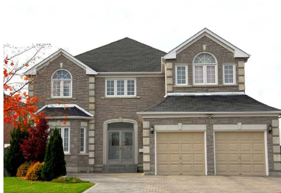
This home design has a prominent garage forward of the main house. The proportions and openings for this home are too small for the overall massing.
