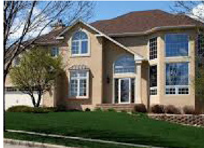
The roof massing and eave at entrance are improperly detailed. Columns and openings are improperly proportioned.
