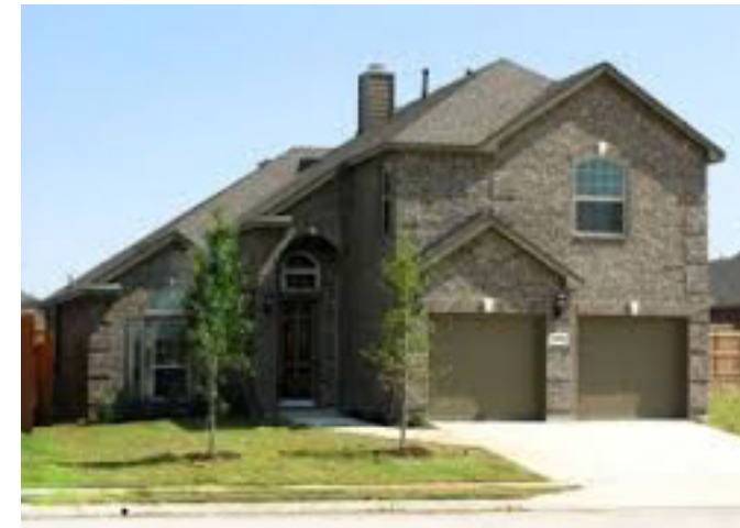
The garage is most prominent and creates disproportioned overall massing. Vent stacks are visible from the street.
