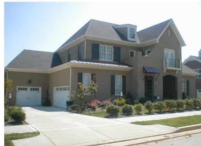
This contemporary Tudor style home has an efficient garage arrangement with a prominent entrance and applied elements.
