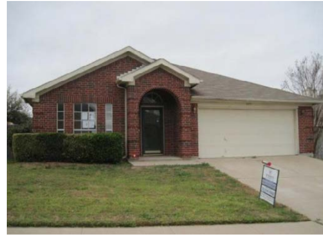
Paired windows are detailed improperly. The garage is too prominent in the elevation.
