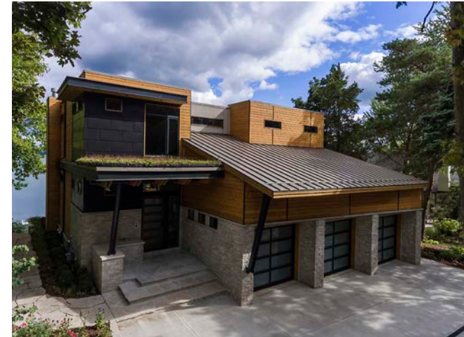
This contemporary home has a monoslope steel roof, exposed structural steel members and flat-topped parapets.
