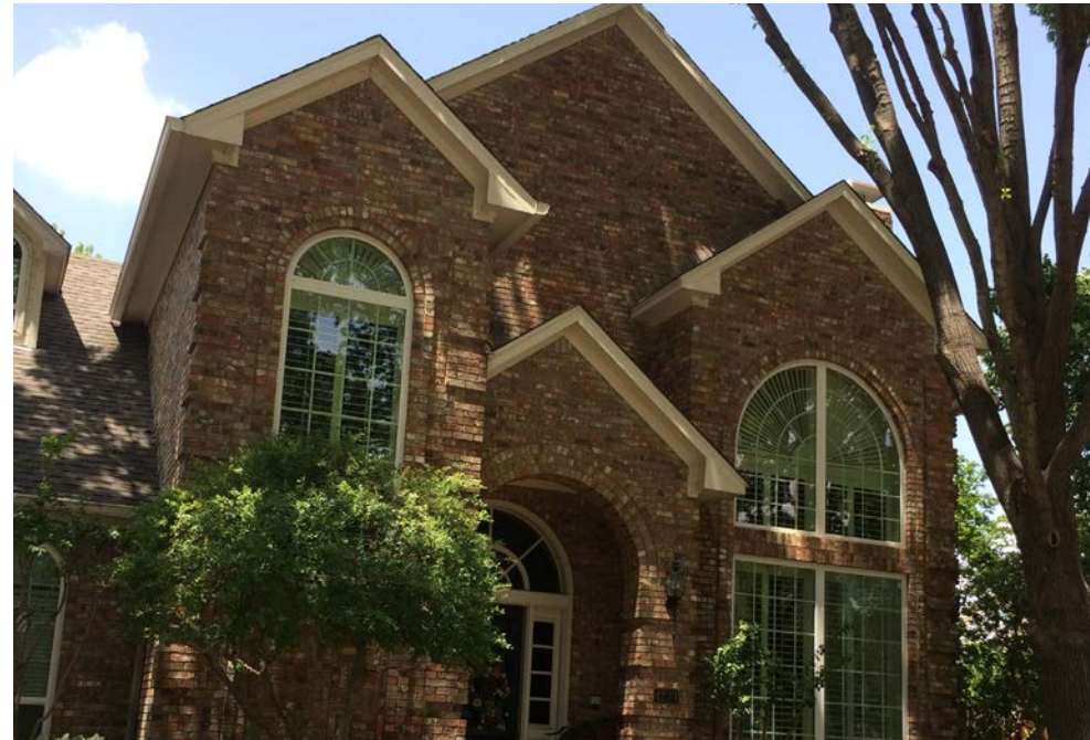
The window openings are too large and out of proportion for the façade. This home has a complex massing where the gable elements are competing for importance.
