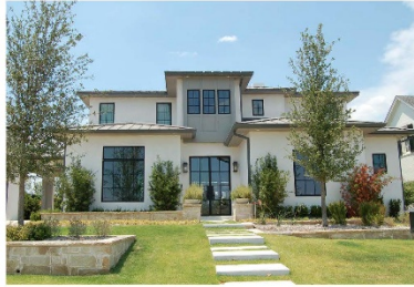
This home design has a garage set back from main house. Entrance is prominent. Massing is more complex with some variation. Minimal detailing is appropriate for the style.
