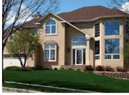
The roof massing and core at entrance are improperly detailed. Columns and openings are improperly proportioned.
