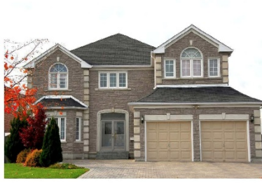
This home design has a prominent garage footprint of the main house. The proportions and openings for this home are too small for the overall massing.
