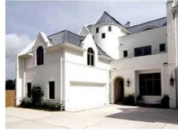
This home has very complex massing with many elements competing for attention.
