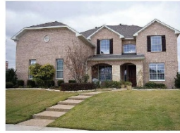
The garage on this home is the largest mass in the elevation. Scaffolds are not sized properly for the openings.
