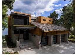
This contemporary home has a monoslope steel roof, exposed structural steel members and flat-topped parapets.
