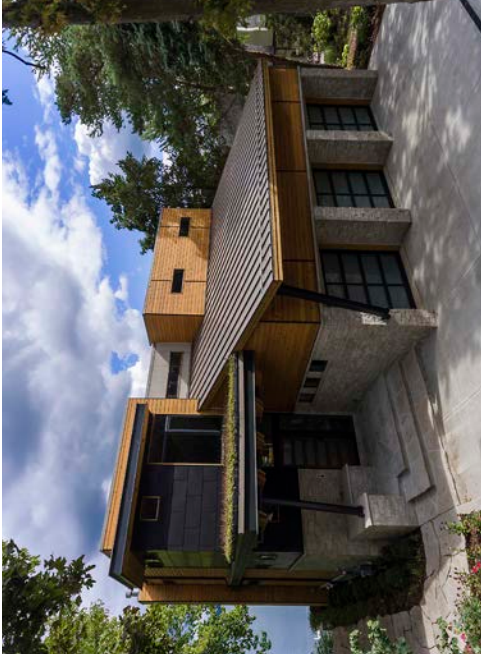
This contemporary home has a monoslope steel roof, exposed structural steel members and flat-topped parapets.
