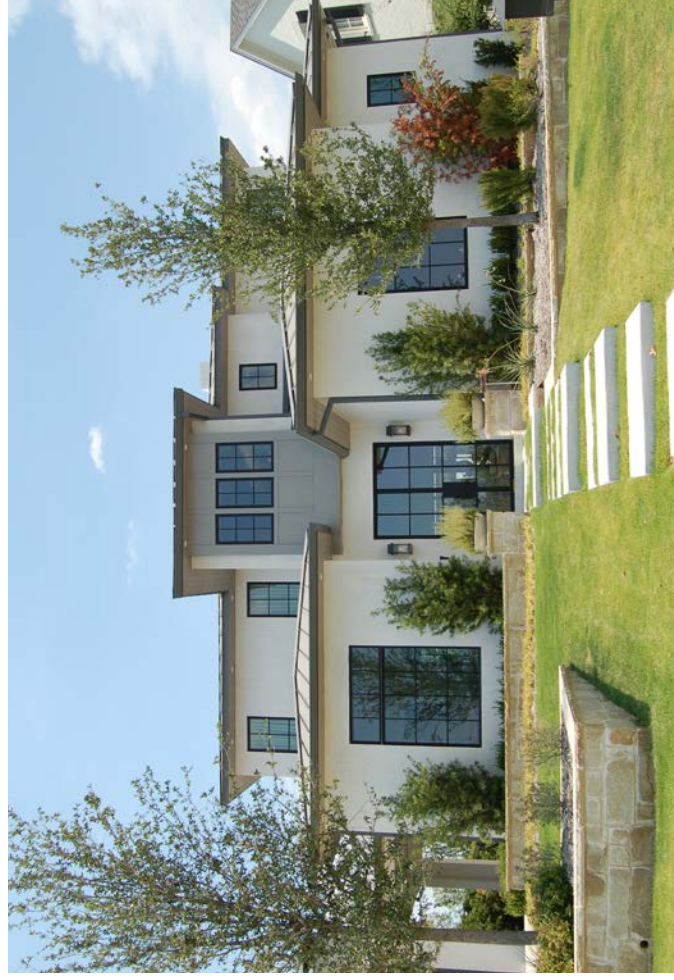
This home design has a garage set back from main house. Entrance is prominent. Massing is more complex with some variation. Minimal detailing is appropriate for the style.
