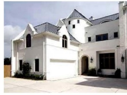
This house has very complex massing with many elements competing for attention.
