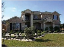
This house has a complex roof and massing. The two-story entrance is disproportionate.
