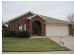
Exterior windows are detailed improperly. The garage is too prominent in the elevation.
