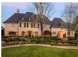
This house has balanced, simple forms that generate a sense of symmetry. Roofs and corners are appropriate for the style.
