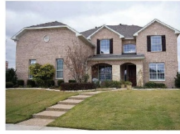
The garage on this house is the largest mass in the elevation. Shutters are not sized properly for the openings.
