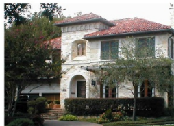
This two-story masonry house has a prominent entry for the style with applied elements for shading from sun exposure.
