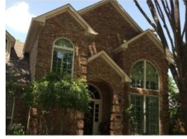
The openings are too large for the home. The massing is too complex for the width of the front façade.
